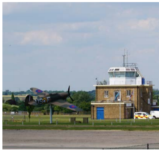
North Weald Airfield, listed control tower
