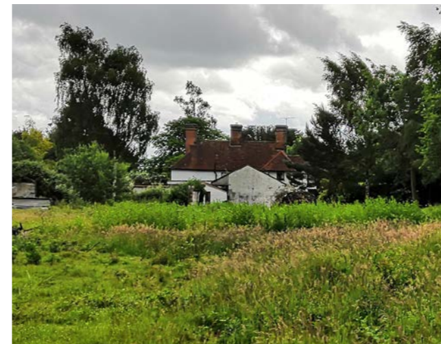
Listed buildings (Tylers Farmhouse)
